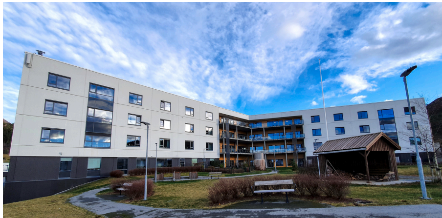
Fig. 1. The pilot building consists of 5 stories, the southern façade.
