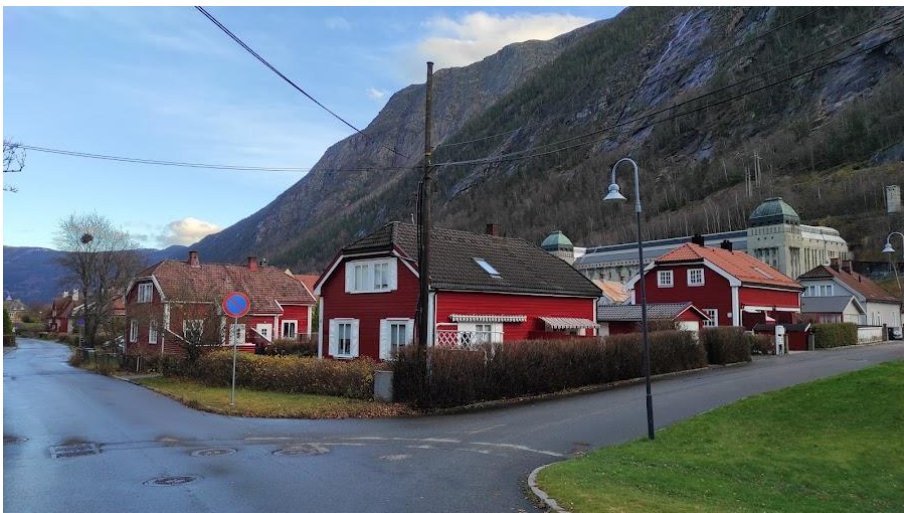
Figure 4.9 Rjukan Company Town with Såheim Kraftverk building as background
