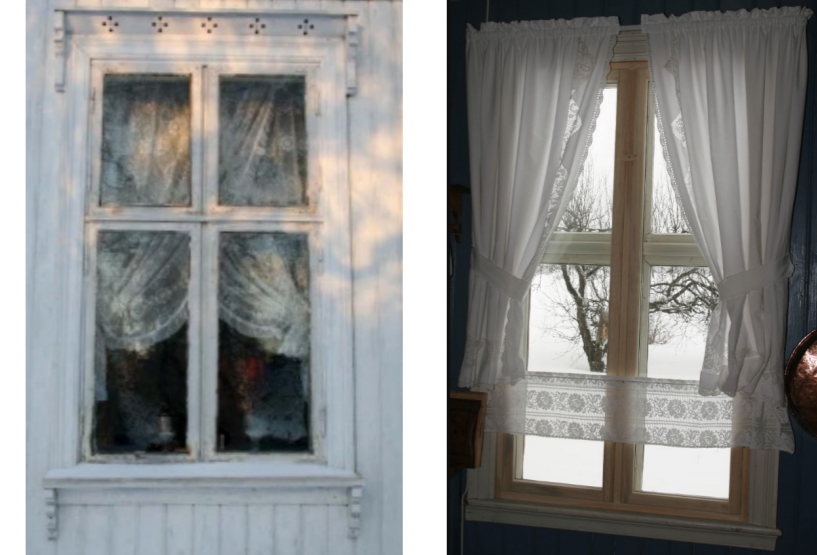
Pictures of the renovated windows (Fjeldheim, 2011).
