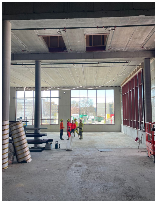
Mechanical workshop, view from 1st floor.
