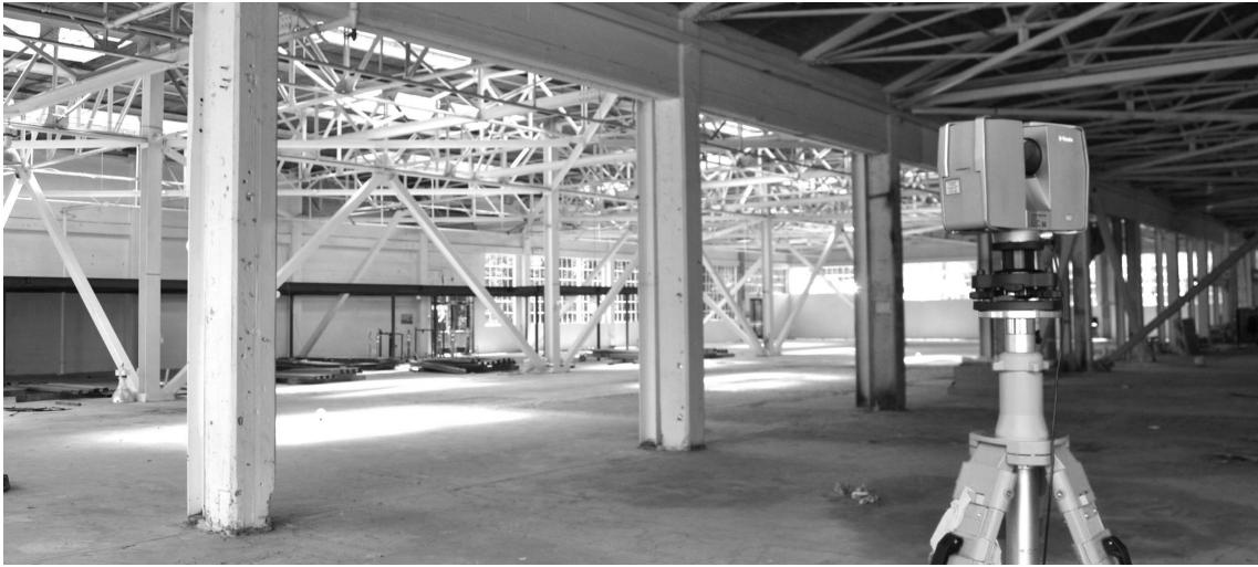
Figure 14: Laser scanning with point-cloud technology. The scanner (right side of the image) is moved around the project and collects coordinates (Meridian Surveying Engineering, Inc., n.d.).
