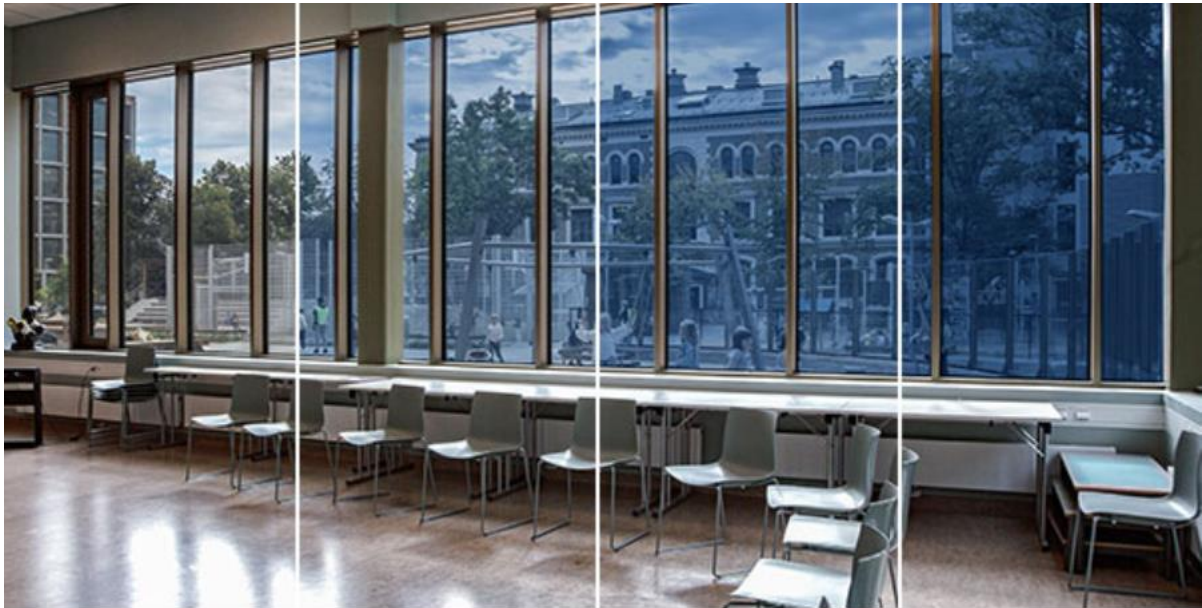
Picture 3: The Electrochromic windows regulate light and heat in the building.
