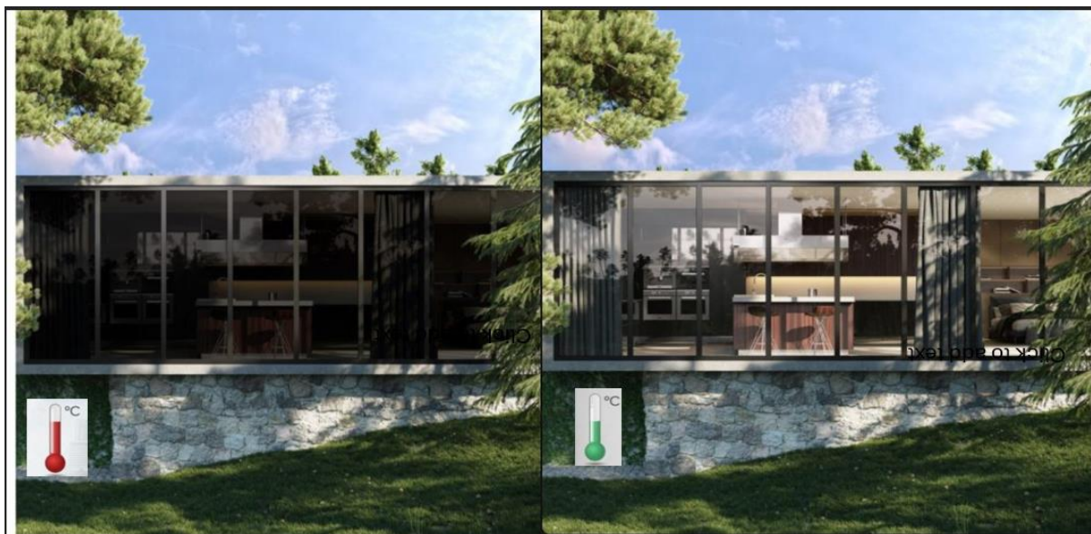
Picture 1: Thermochromic smart windows reacting to temperature fluctuations.
