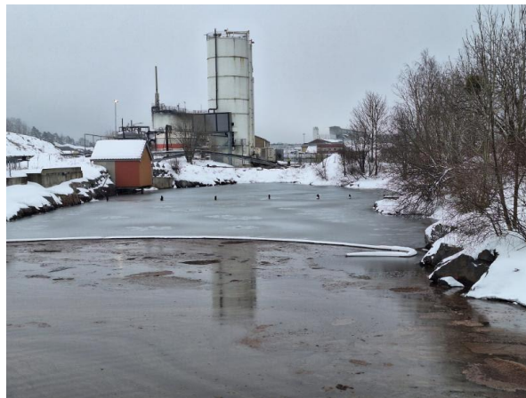
Figure 1: The precipitation and sedimentation pool at the wastewater treatment plant at Langøya.
