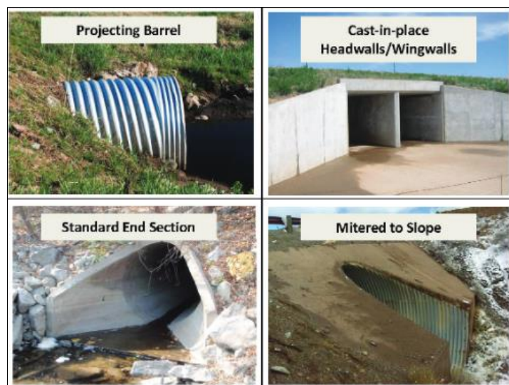
Figure 1-2: Standard Inlet Types (Schall et al., 2012).
