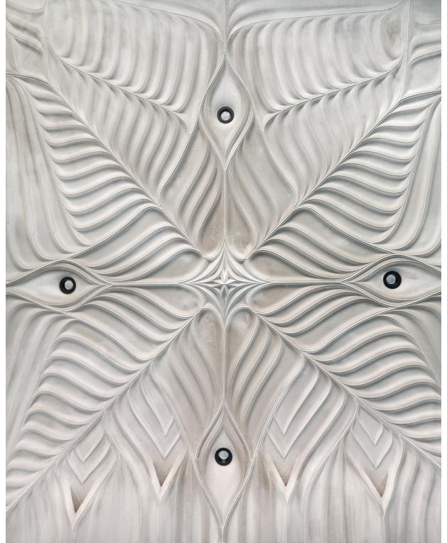
Figure 2: View of the lightweight floor with integrated TABS and ventilation system in office 2, the four air outlets are at the bottom. Photo: Roman Keller.
