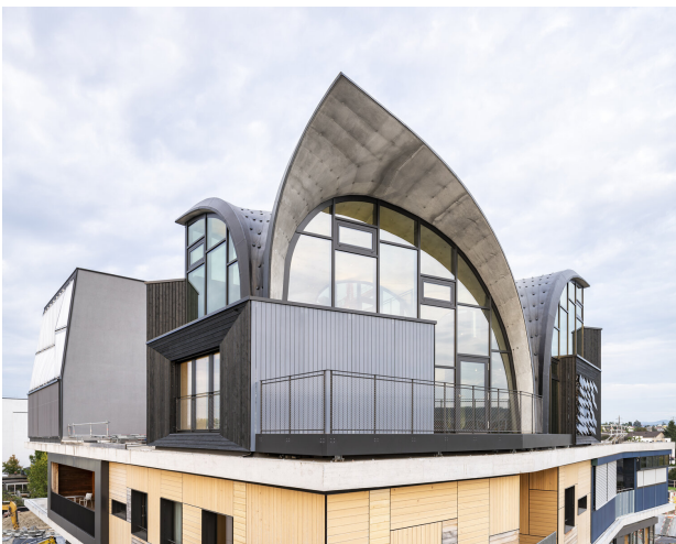
Figure 1: External view of the HiLo unit from the south-west. Office 1 is located on the HiLo bottom floor.
