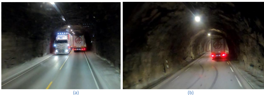
Figure 7. (a). Tight passage when encountering oncoming truck. (b). Narrow tunnel without centerline. Both seen from truck 3.
