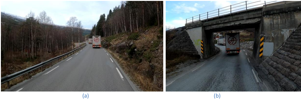
Figure 8. (a). Narrow rural road (b). Narrow railway underpass in curve with limited sight distance. Both seen from truck 3.
