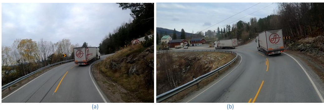
Figure 6. (a). 16-meter radius hairpin in steep 6.2% uphill (b). 80-meter left-turn in a slight downhill. Both views seen from truck 3.
