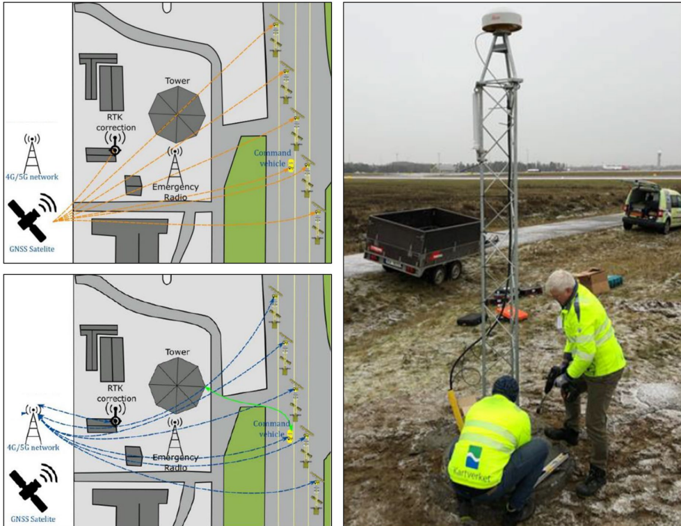
Figure 21: GNSS and communications ( left ), and CPOS base station ( right ) at Avinor.
