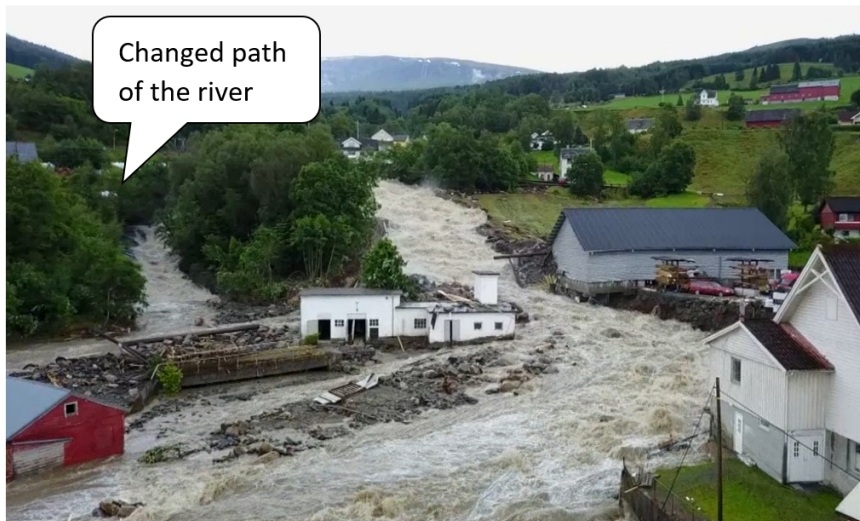
Figure 1.1: Changed path of the river during the flash flood. Source: tv2.no.
