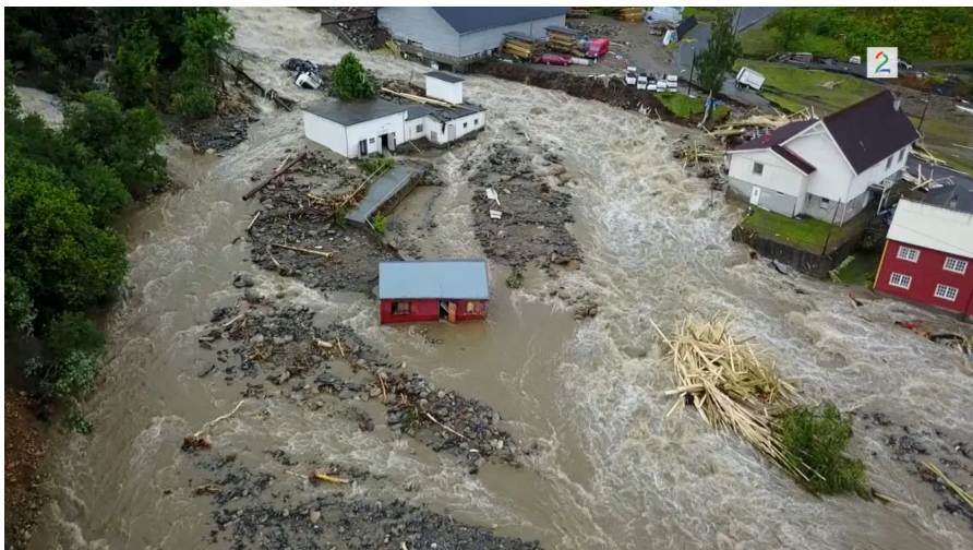
Figure 1.2: Debris and damage in Utvik during the flash flood. Source: tv2.no.
