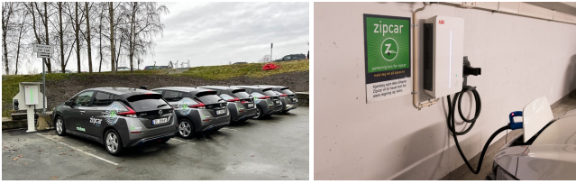
Figure 3: Deployed shared EVs in an outdoor location, and in a parking garage with a V2G charger (from [23], photos by Trondheim kommune)
