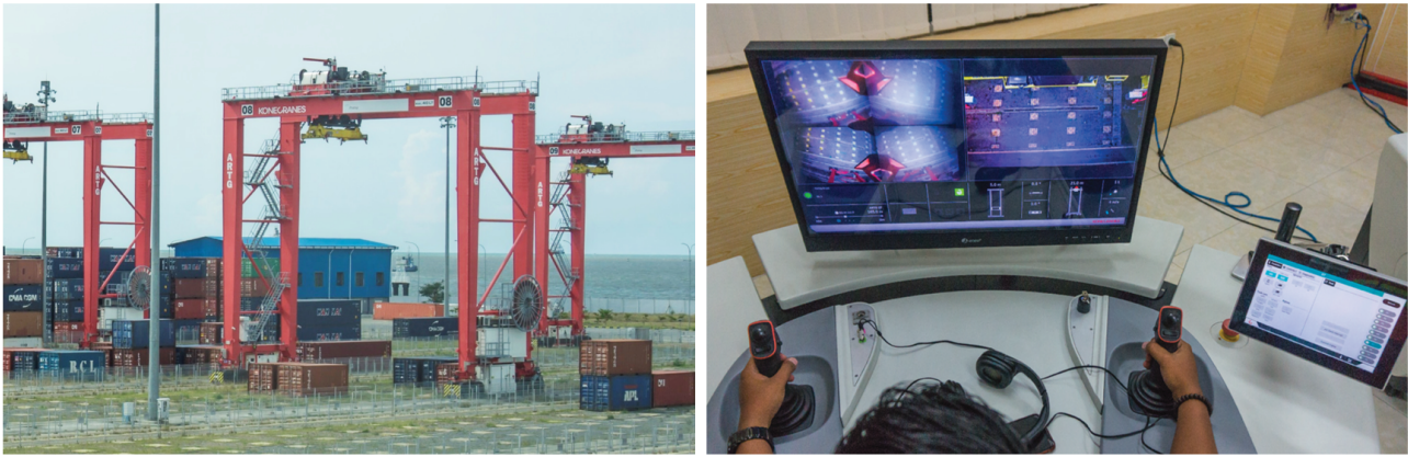
Figure 1: The left image shows the example of RTG cranes that can be operated remotely. The right image shows the remote control station used by the operator to operate any RTG cranes within one port.
