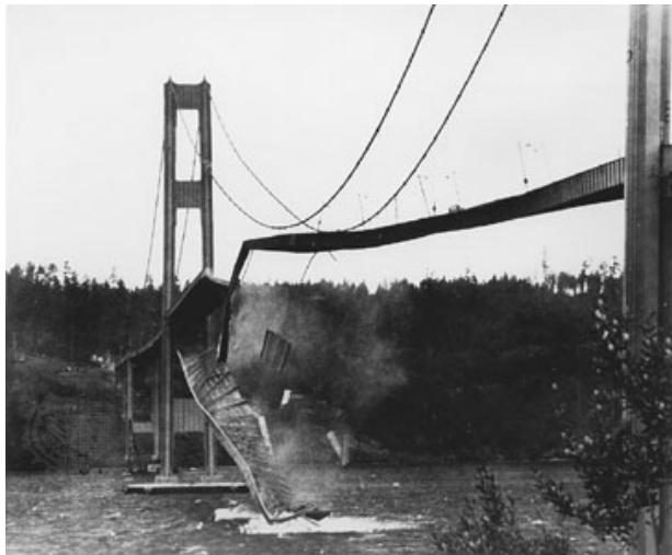
Figure 3.5: Tacoma Narrows Bridge collapsing, November 7, 1940 [26]
