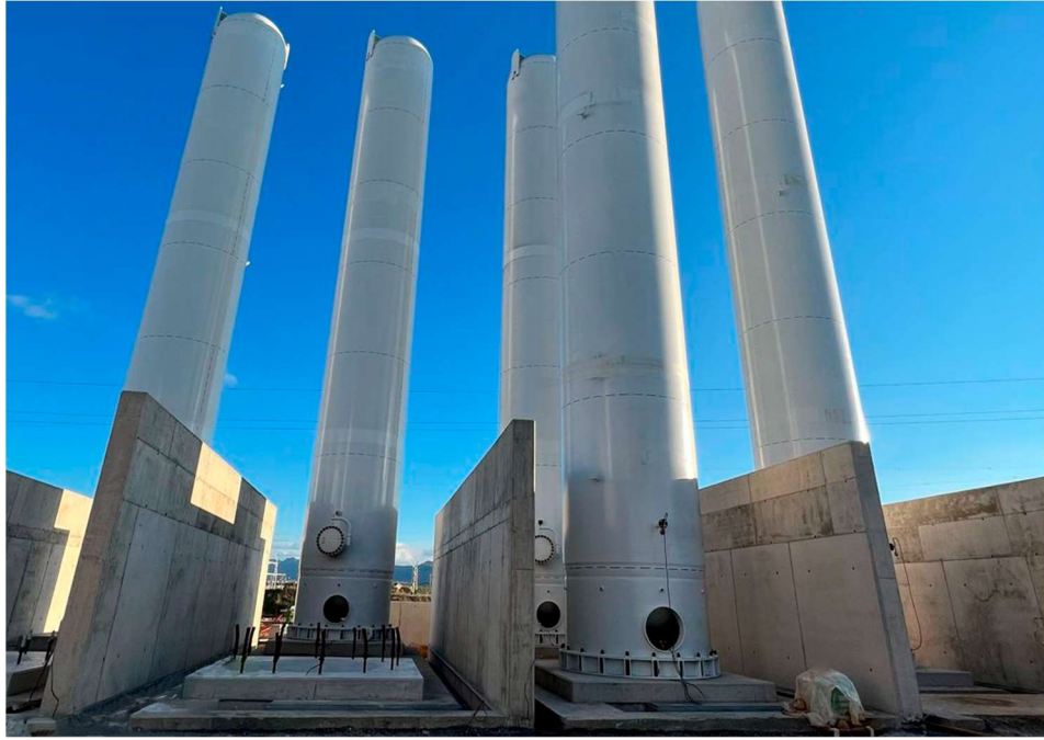
Figure 2-20: Five H 2 Tanks by Iberdrola. 237 MWh (HHV) capacity for each tank. Image Credit: Idesa.net [89]
