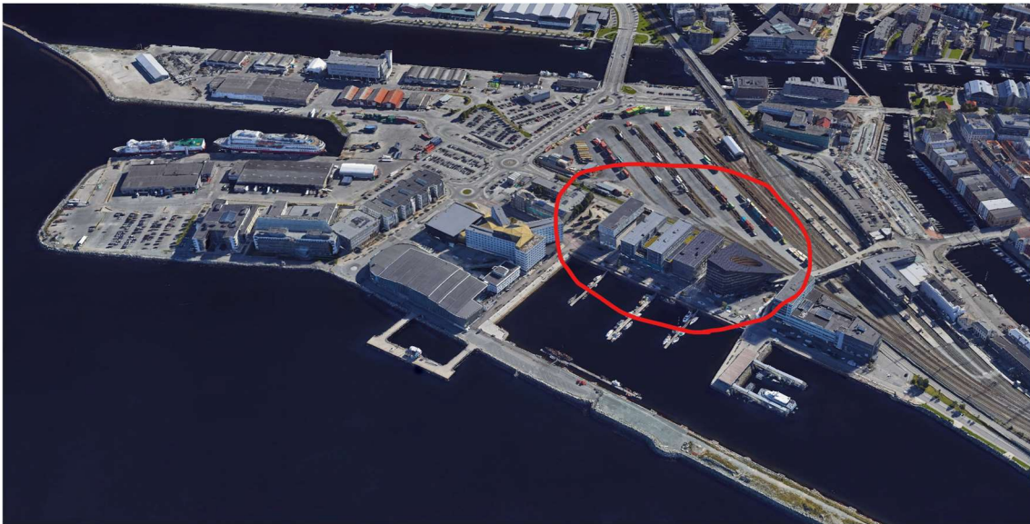
Figure 5-3: The building group with the 0.9 GWh/year heat demand as of 2024. Express boat terminal seen to the lower right-hand side in the marina. Image Credit: Google Maps
