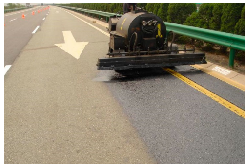
Figure 2. Fog seal technology with operation.
