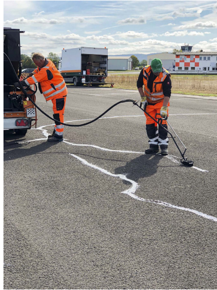
Figure 1. Hot pouring technology to heal the cracks.
