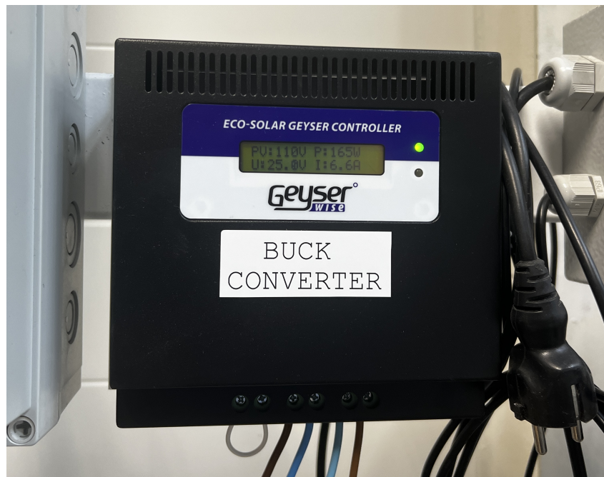
Figure 3.1: The Geysewise ECO MPPT solar charge controller. 72V & 48V model are in equal housings.
