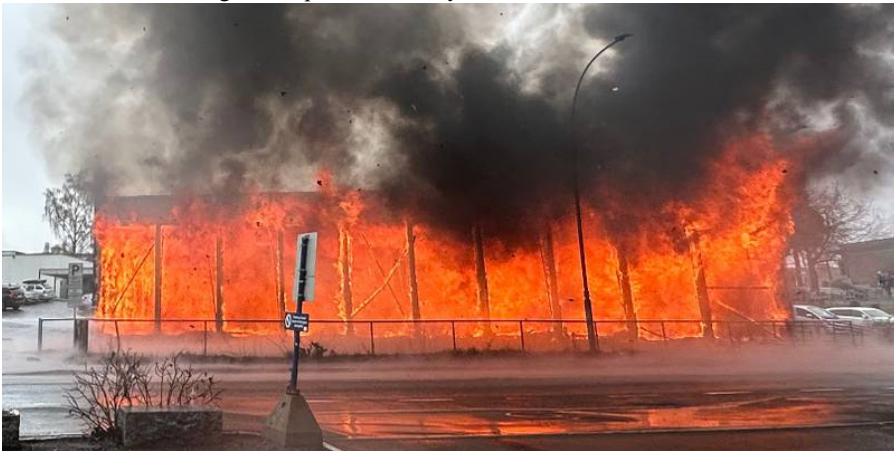
Fig. 69 Massive fire at Lambertseter school gym. Here, all windows have been broken. The image was taken approx. 16 minutes after ignition. Photo: Glenn Berggren, used with permission.
