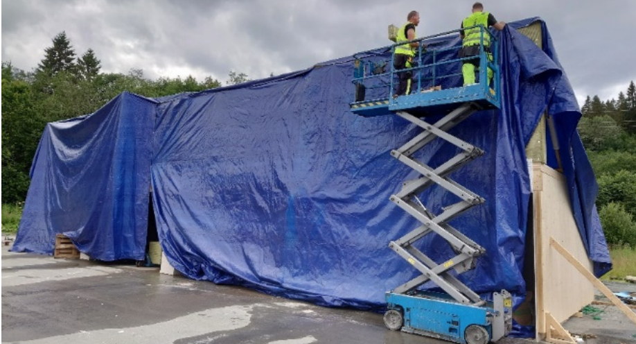
Fig. 50 The compartment was protected against rain with several large tarps.
