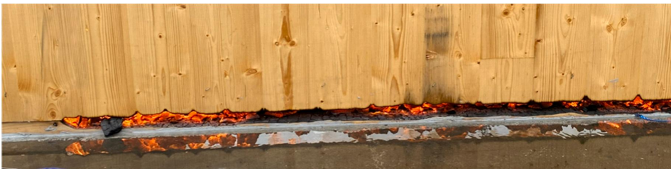
Fig. 31. The fire burned through the intersection between the back wall and the bottom plank at approximately 60 min. The image is taken at a later point when the gap had become larger. The lack of a fire sealant between the bottom plank and the CLT wall enabled this and highlights that connection details are crucial to fire safety.
