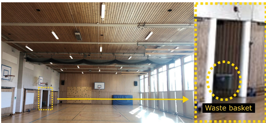
Fig. 70 Image of Lambertseter school gym before the fire. The fire started in a waste basket similar to the one highlighted. The location was in another entrance corridor more to the left of the image perspective. The image is edited with permission by SG AS [109].
