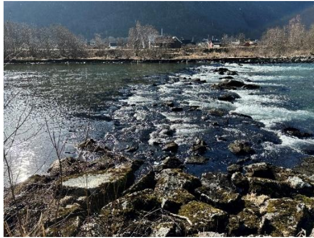
Figure 2. 1 weir at øye
