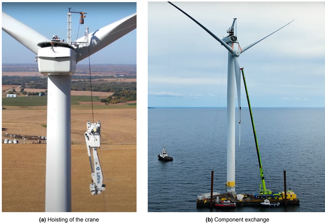
Figure 2.7: A component exchange using a self-hoisting crane [28]
