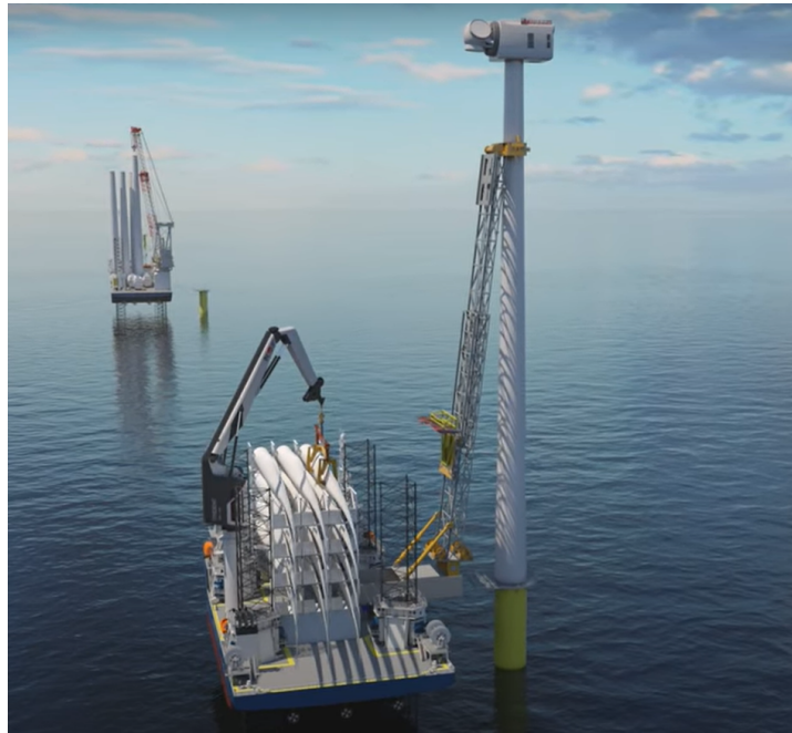
Figure 2.11: A gripper frame for blade installation, with a supporting crane and a transferable yoke (Image courtesy of NOV)
