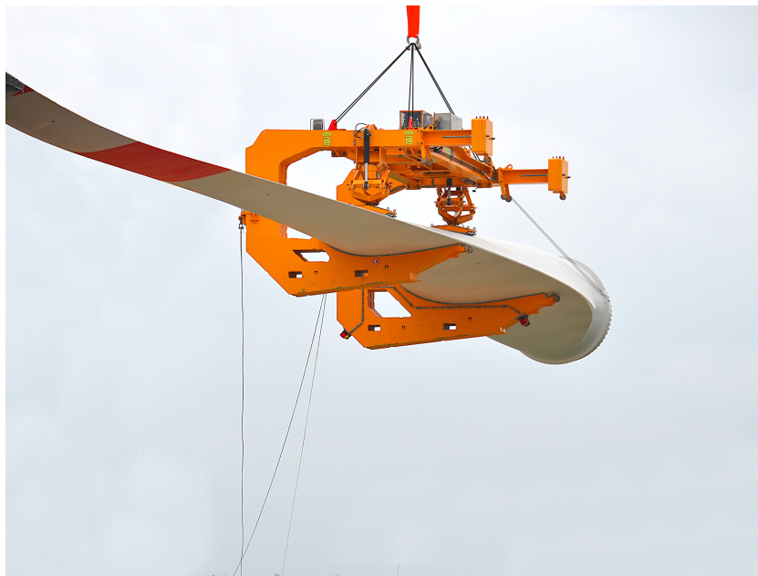
Figure 3.3: A yoke is used to grab and lift a blade
