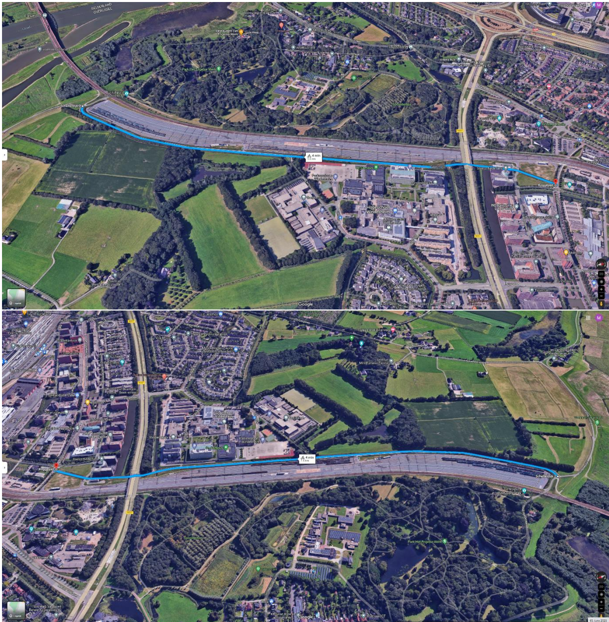
Figure 40. Overhead views of section 4. Photo credit: self
