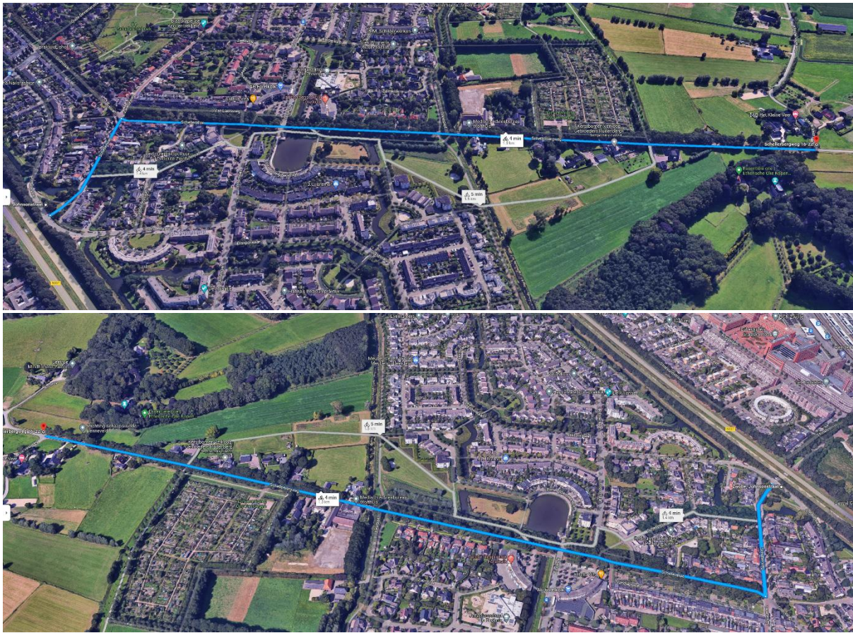
Figure 33. Overhead views of section 2. Photo credit: self
