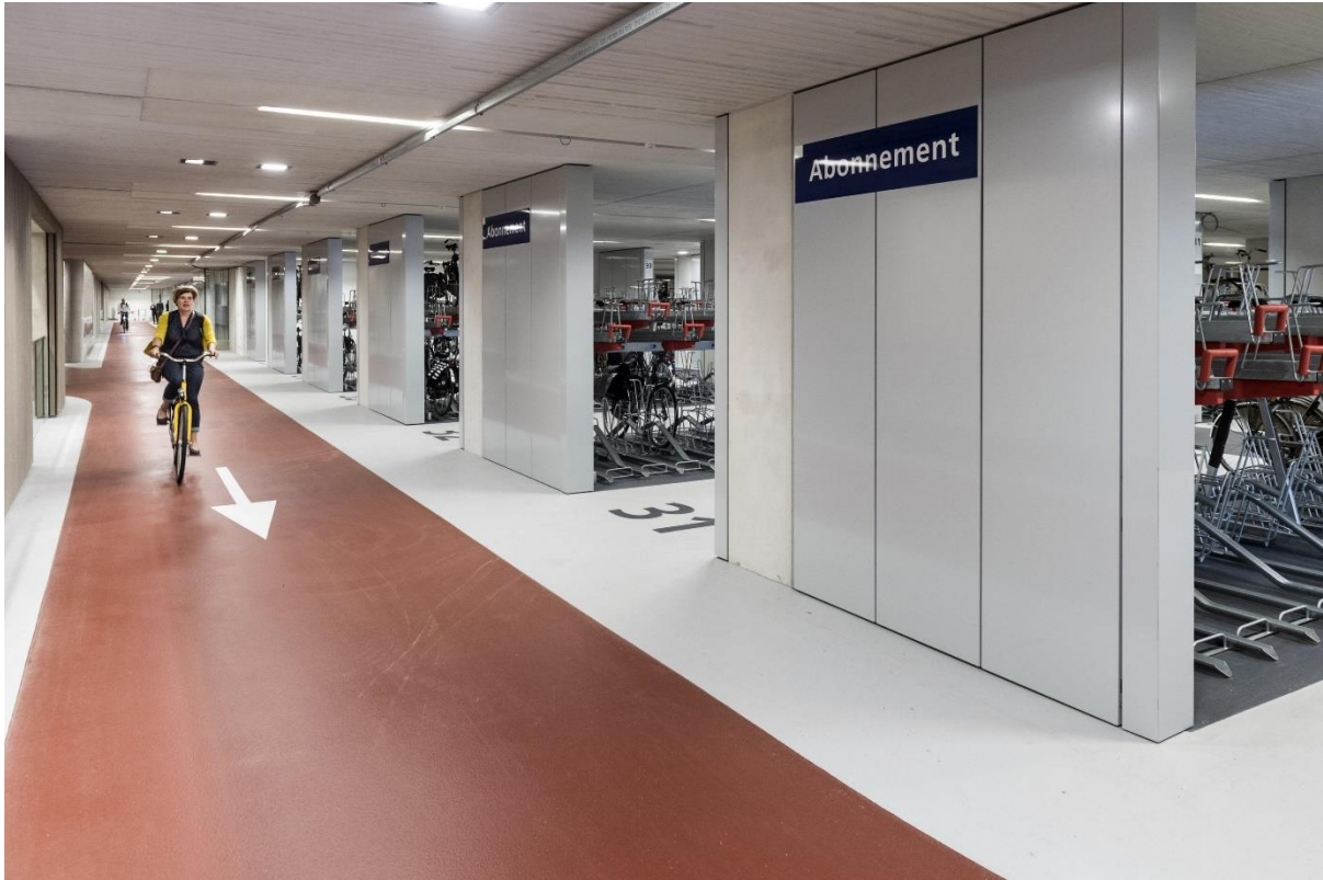
Figure 12. The world's largest bicycle parking garage in Utrecht Central Station. This infrastructure helps to solidify the bicycle as a marker of Utrecht's sense of place. Source: /u/gahte3 Reddit, 2019.
