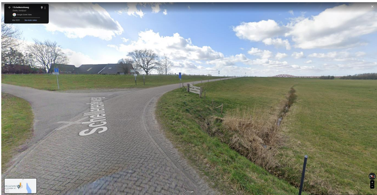
Figure 38. On street perspective of the transition zone up onto the dike in Section 3 Photo credit: Self (2023) via Google maps. Image captured March 2023.
