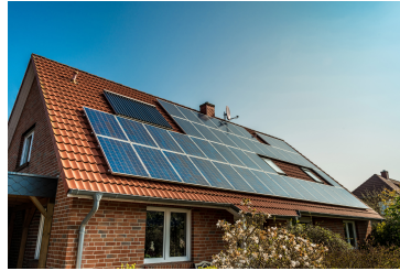
(b) Solar panels on a house [7]
