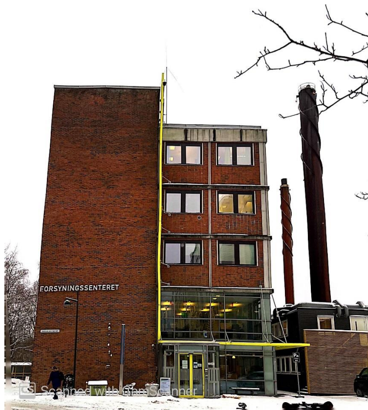
Figure 9: The supply center
