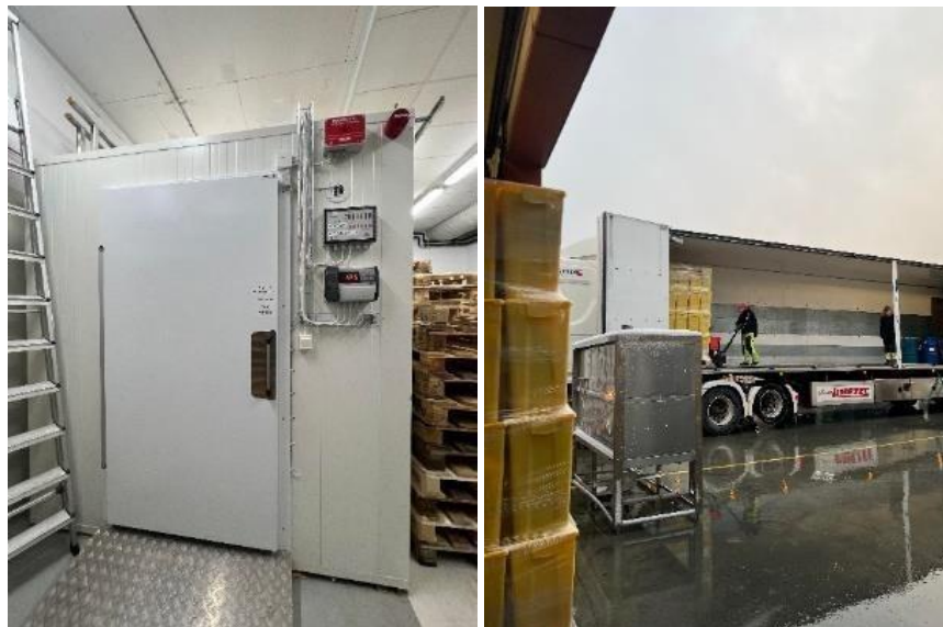
Figure 16: Storage and transport of hazardous waste
