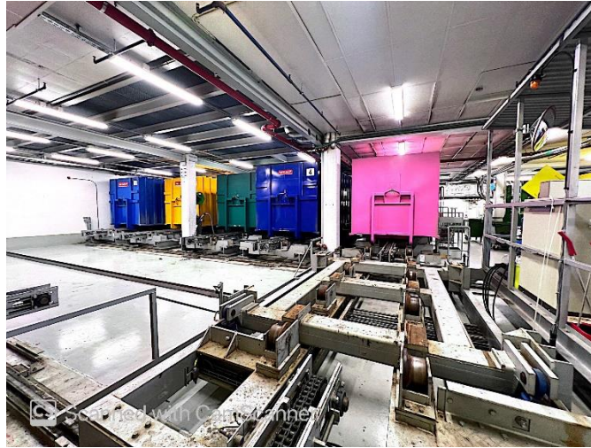
Figure 13: Waste treatment facility
