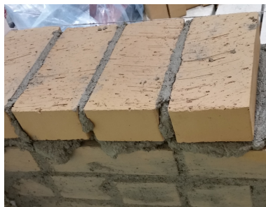
Figure 2. Close-up of bricks during brick laying.
