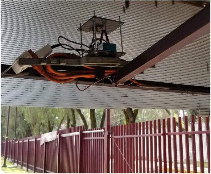
Fig. 7. UPIITA station installation
