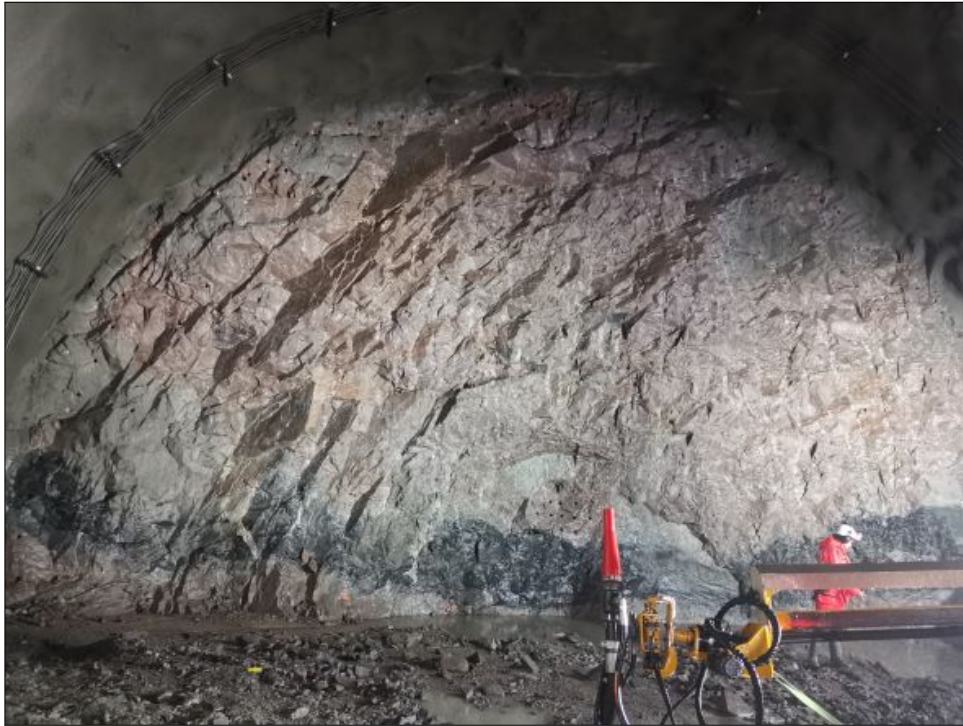
Figure 8.1: Amphibolite with a dyke-like appearance in the gneiss. The amphibolite dips steeply 70 degrees into the tunnel face. The picture is taken at the Kleverud tunnel face.
