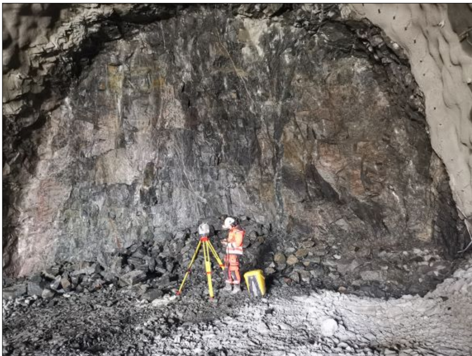
Figure 8.2: Strongly tectonized vertical amphibolite dyke with surrounding gneiss. The Picture was taken at the Espa tunnel face.
