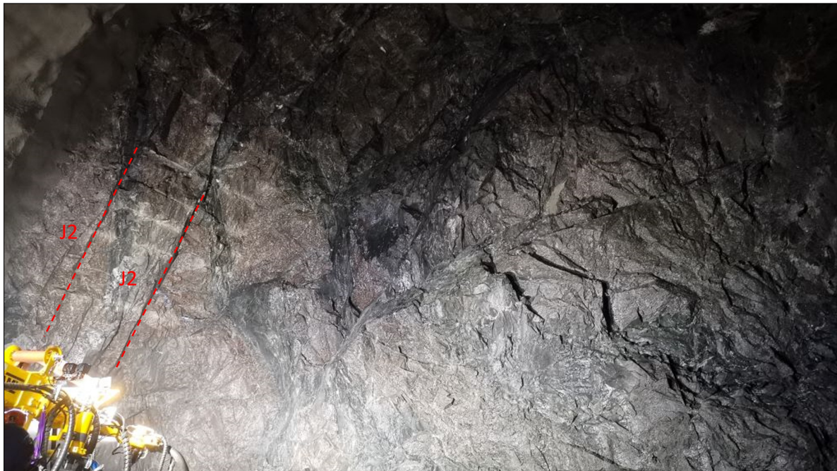
Figure 8.6: J2 joint set visible in the gneiss on the left-hand side. Joint spacing 0.5-3 m
