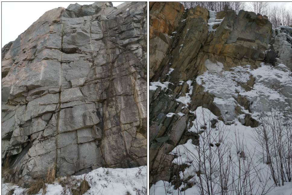
(a) Example of the sub-horizontal joint set J3 in a gneiss rock cut south of Kleverud. (b) Example of joint set J1 in a gneiss rock cut south of Kleverud.
