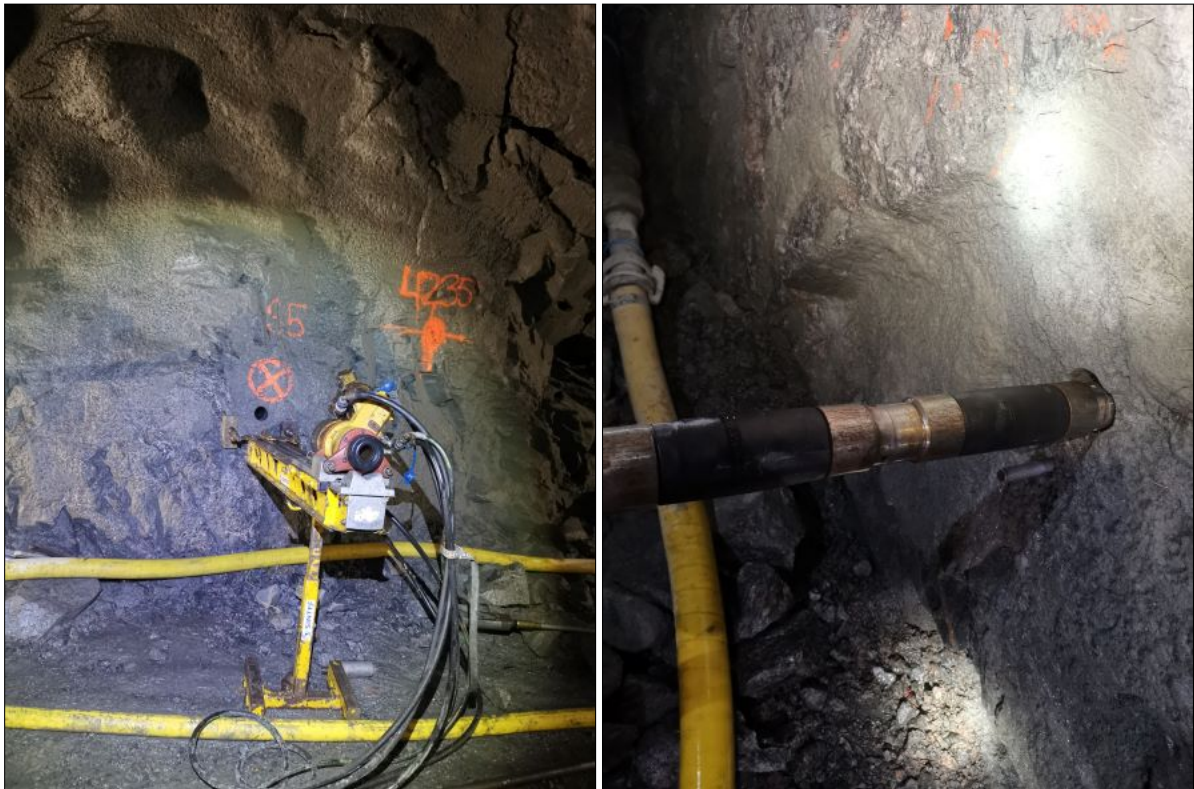
(a) Setup of the drilling of rock cores and holes (b) Setup of the double packers with a 15 cm test section later used for WPT.
