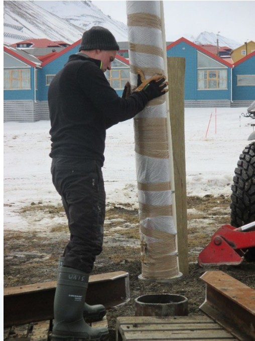
Fig. 10 Pile installation
