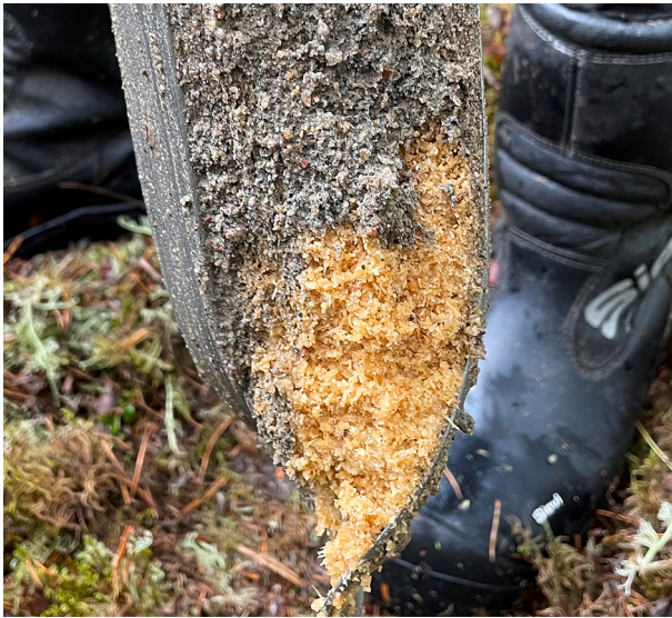
Fig. 12. Photograph of sawdust and sand in auger extracted from Site 1 Embankment II in May 2021
