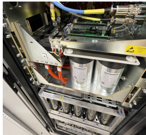
FIGURE 10 Photograph of the laboratory setup, showing the power stack, gate drivers and DC-bus filter capacitors integrated into the cabinet. The storage capacitors can be seen at the bottom.
