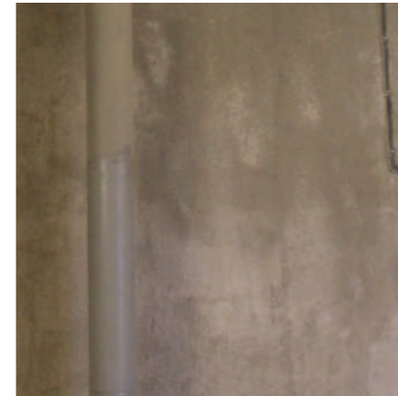
INTERNAL CONCRETE WALLS IN THE SILOS
