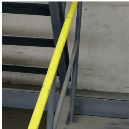
PAINTED STEEL RAILING IN THE SQUARED SILO
