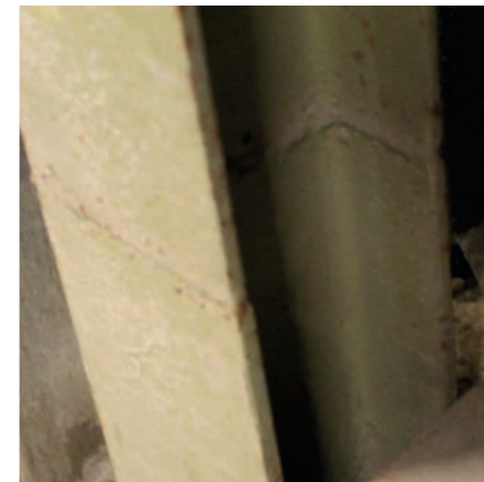
PAINTED STEEL FRAME IN THE STORAGE HALL
