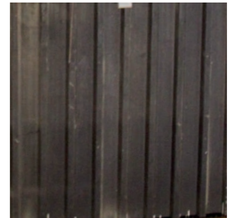
CORRUGATED IRON IN THE STORAGE HALL
