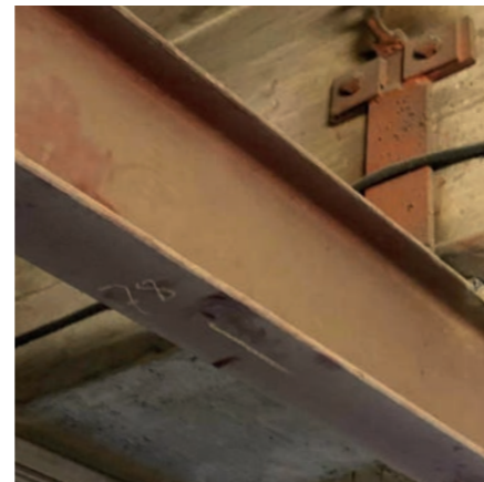
PAINTED STEEL BEAM IN THE SQUARED SILO
