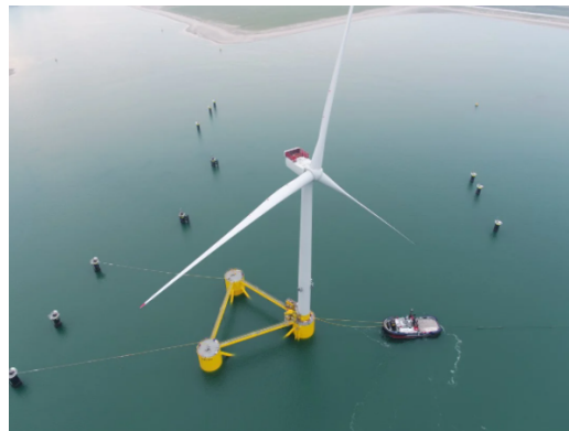
Figure 28: Storage of the Kin04 floater with horizontal mooring lines and bollards (Buljan, 2022b)
