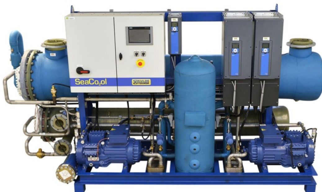
Figure 18: RSW system based on CO 2 developed by Kuldeteknik AS ( Kuldeteknik AS, 2011 )
