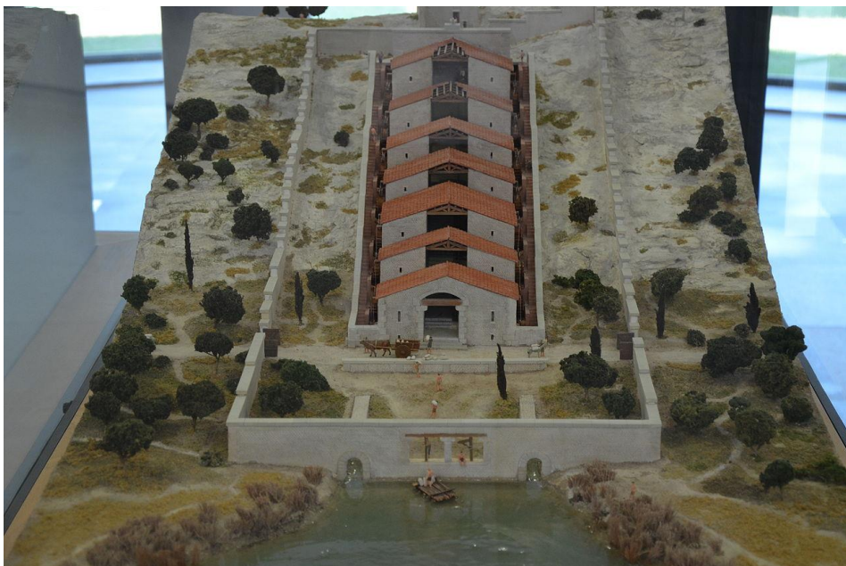
Figure 1 - Barbegal Mills - a cascade of 16 overshot watermills built by Romans in the 2nd century. Source: Carole Raddato, Museum of Ancient Arles, Arles, France.
