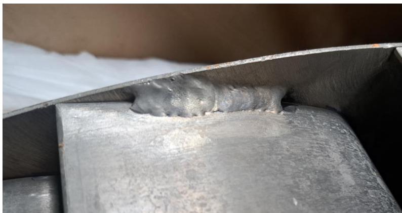
Figure 36 - Spot welds used to fix the buckets to the wheel, causing minor leaks in between the buckets and wheel's walls
