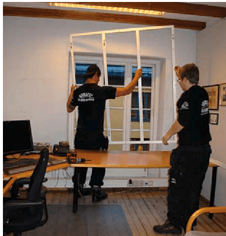
Fig. 3.1. Installation of a secondary glazing improving the window's U-value from 4.6 W/(m 2 K) to 1.6 W/(m 2 K). Photo: Marte Boro [125].
