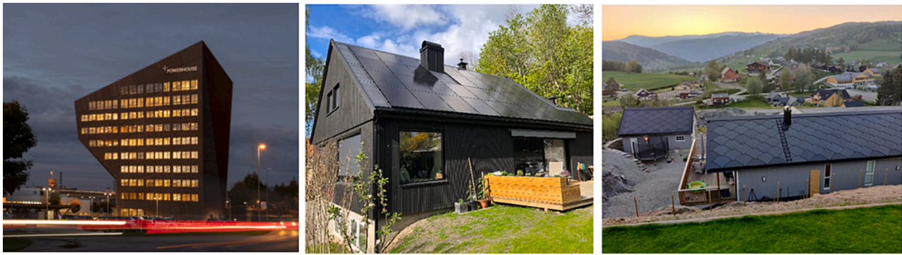
Fig. 5.4. Powerhouse Telemark (left) [77]. Two Norwegian houses with BIPV roofs (middle and right) [16].
