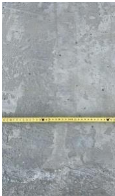
g) Top surface of the impact area after first impact
