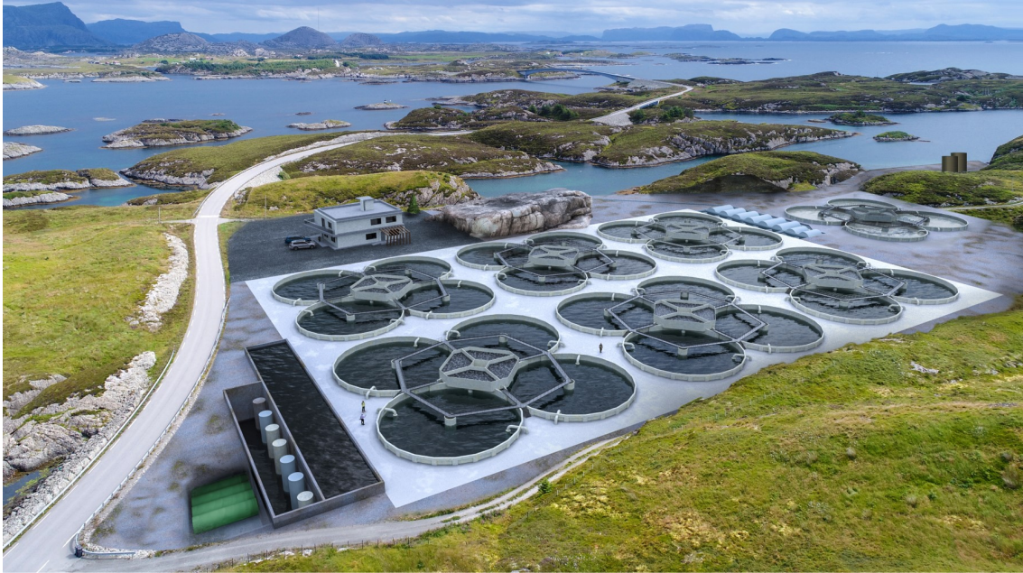
Figure 7.1: An illustration of the production facility with seven modules, where each module contains four tanks
