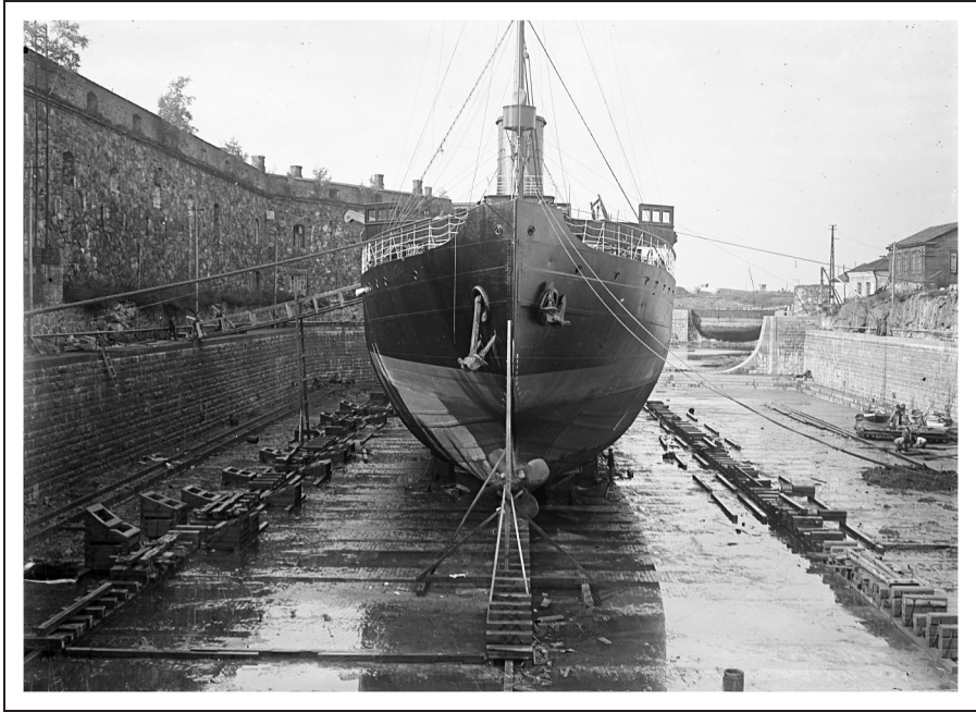
Figure 1. Icebreaker Wäinämöinen (formerly Tsar Mikhail Feodorovich , later renamed Suur Töll ) at Suomenlinna dock around 1920, showing the ‘American-type’ bow.
