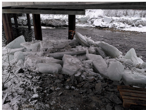
Fig. 1. Shear wall and stranded ice floes surrounding the piers of Sokna bridge after an ice run at the end of the 2019–2020 winter season.
