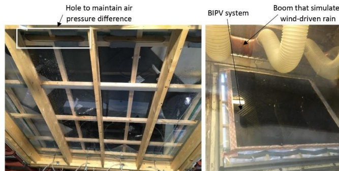
Fig. 11. BIPV system 1 during wind-driven rain testing in the RAWI box. Interior BIPV side (left) and exterior BIPV side (right).
