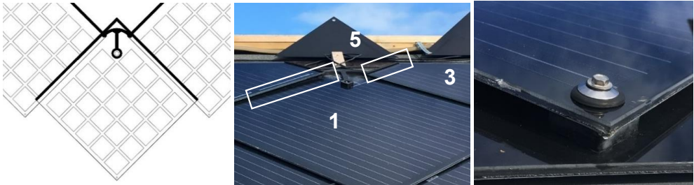
Figure 42. Rubber element on upper part of the solar shingle (schematically shown on the drawing to the left and how they are attached on the real roof shown on the photo in the middle) and (right) lower part of the solar shingle. 1 – basic solar shingle, 3 – solar shingle top and 5 – matching glass-glass triangle element on an actual building roof (photo and drawing by Anna Fedorova).
