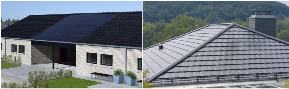
Figure 47. BIPV system with horizontally orientated modules integrated with metal roof plates on the left. Steel roof plates installed on an actual building roof on the right [127,128].
