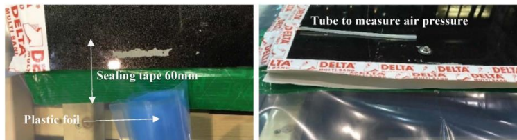
Fig. 5. Sealing the edges of the BIPV system using sealing tapes and polyethylene foil (view from the frontside). On the right photo a tube used to measure the differential air pressure is visible lying on the black module. Study 3 (Table 3).
