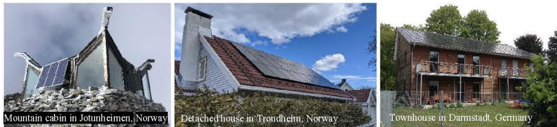
Figure 1. Off-grid PV system installed on the façade of a mountain cabin, building applied PV (BAPV) system attached on the roof tiles, PV tiles system (BIPV) integrated into the roof. (Source: authors’ photos)
