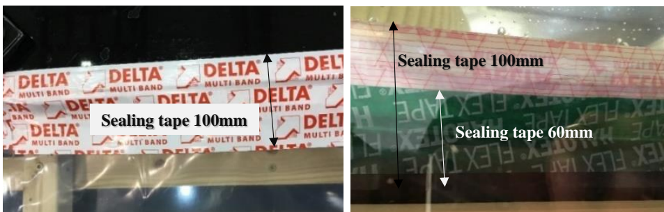
Figure 36. View of a complete taping from the frontside (left) and from the backside (right) [116].
