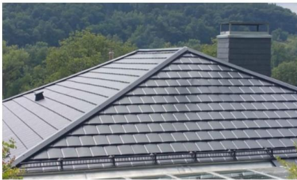
Fig. 9. Isola Powertekk steel roof plates (non-PV) installed on an actual building roof (" https://www.isola.com/ ").
