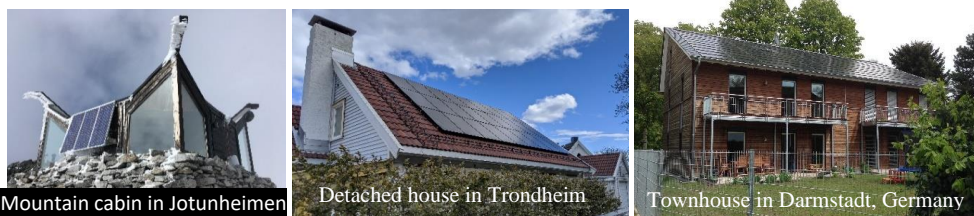
Figure 1. (left) Off-grid PV system installed on the façade of a mountain cabin, (middle) building-applied PV (BAPV) system attached on the roof tiles and (right) PV tiles system (BIPV) integrated into the roof. (Photos by Anna Fedorova and Bozena Dorota Hrynyszyn) [14].
