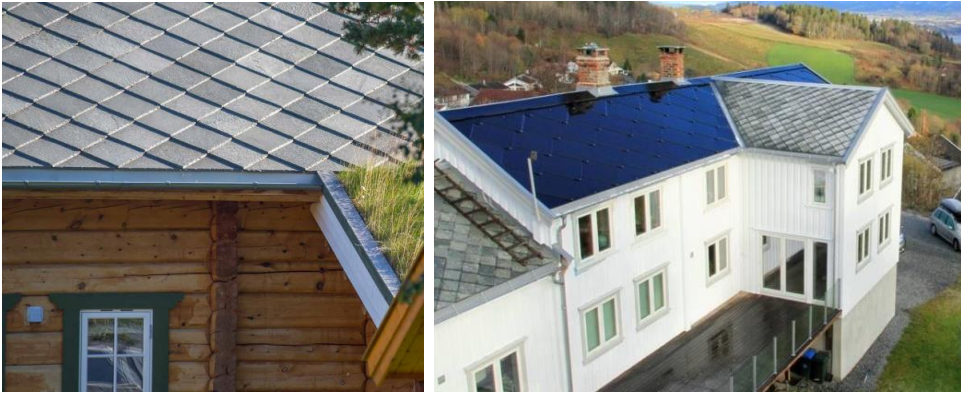
Figure 10. (left) Example of traditional slate roofing tiles [34] and (right) solar shingles installation along traditional slate roofing tiles [35].
