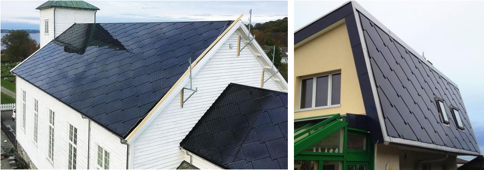
Figure 11. Solar shingles installed on pitched roofs [25].
