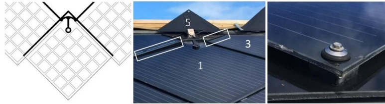
Fig. 5. Rubber element on upper part of the solar shingle (schematically shown on the drawing to the left and how they are attached on the real roof shown on the photo in the middle) and lower part of the solar shingle (right). 1 – basic solar shingle, 3 – solar shingle top and 5 – matching glass-glass triangle element on an actual building roof.
