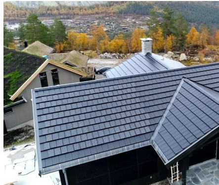
Figure 13. (left) Solar tile made of a ceramic material [37] and (right) their installation on a roof [38].
