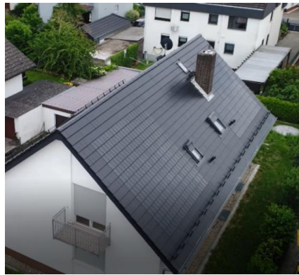
Figure 14. (left) Solar tile made of a concrete material and (right) their installation on a roof [39].
