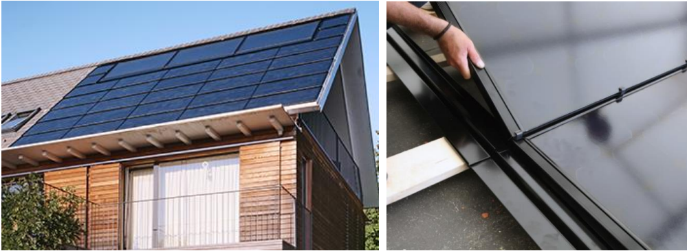
Figure 6. Examples of in-roof mounting BIPV systems [28].
