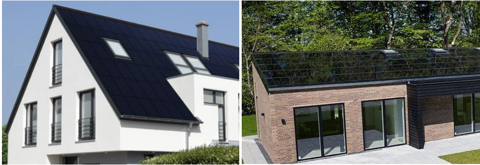
Figure 46. (left) BIPV system with vertically orientated modules and (right) horizontally orientated modules installed on an actual building [127].
