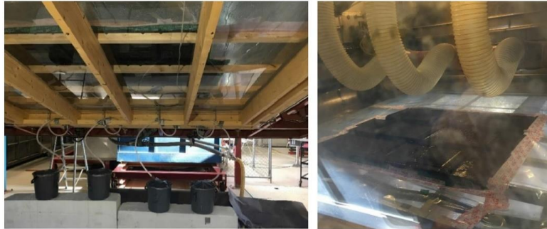
Fig. 15. BIPV system 2 during wind-driven rain testing in the RAWI box. Interior BIPV side (upper photo) and exterior BIPV side (bottom photo).
