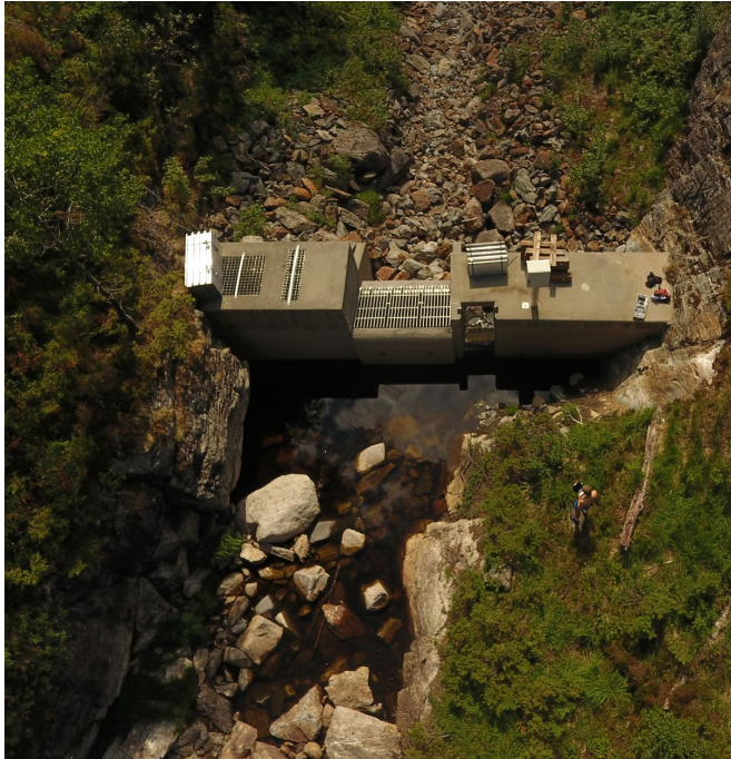
Figure 1. Downstream view of Stigansåni secondary intake during dry conditions.
