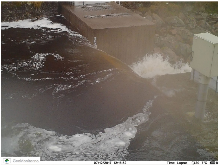
Figure 2. Stigansåni secondary intake during wet conditions.
