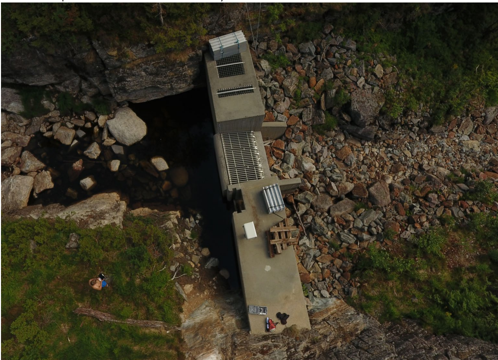
Picture: Side view of Stiansåni secondary intake
