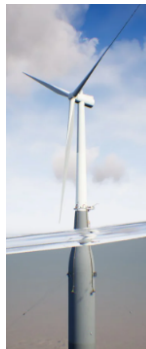
Figure 2.8: Hywind Tampen spar concept Source: (Aker Solutions 2021)
