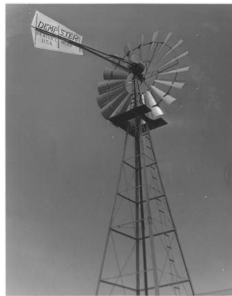
Figure 2.2: Steel blade windmill for water pumping, Midwest - US Source: National Park Service (2019)
