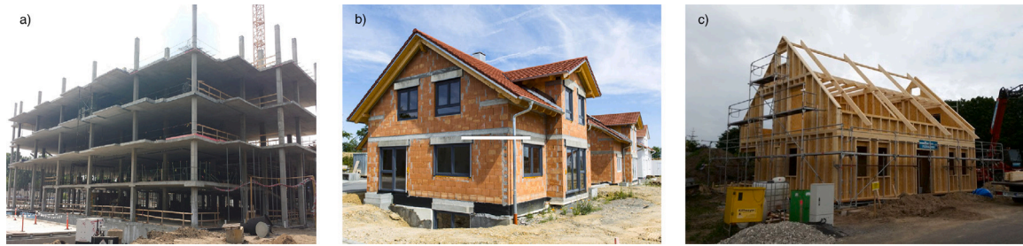
Fig. 2. Typical structural types for German residential buildings: Reinforced concrete structures (RCS); (b) Masonry structures (MS); (c) Timber structures (TS).
