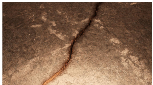
Figure 3.35.: Rendered image of a crack with a Crack Width of \simeq 10mm .
