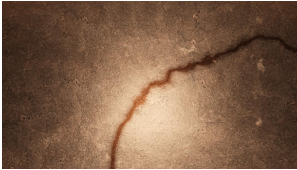
Figure 3.12.: Rendered image of a crack with a Noise Texture W of 0.
