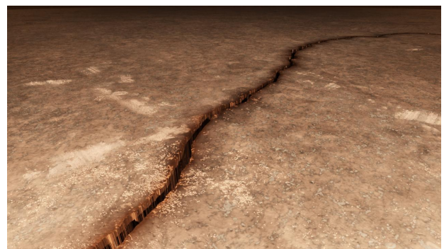
Figure 3.41.: Rendered image of a crack with a Crack Edge Height of 10mm .
