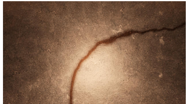
Figure 3.27.: Rendered image of a crack with a Noise Texture Roughness of 0.55.
