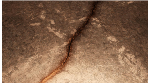
Figure 3.45.: Rendered image of a crack with a Corrosion Spread of 150.
