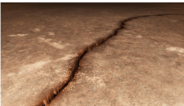
Figure 3.40.: Rendered image of a crack with a Crack Edge Height of 5mm .
