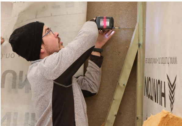
FIGURE 111. Addition of extra cross-bracing
