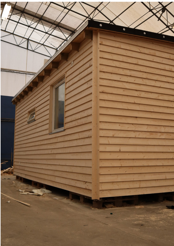
FIGURE 121. Trim is added to edges of exterior cladding
