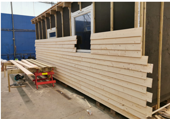
FIGURE 117. Exterior cladding prior to being cut to size
