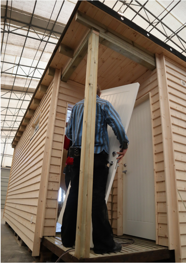
FIGURE 124. Door frames are built, and doors installed
