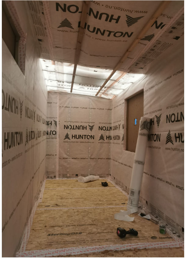
FIGURE 112. Vapour barrier added to the ceiling and roof construction begins
