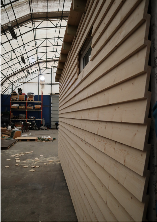
FIGURE 120. Exterior cladding completed
