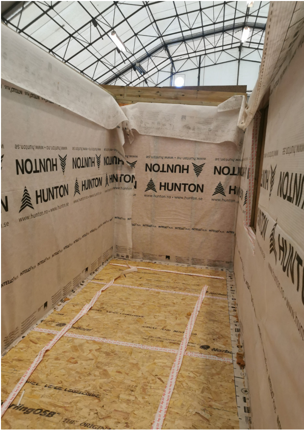
FIGURE 109. Walls standing and fixed to the floor
