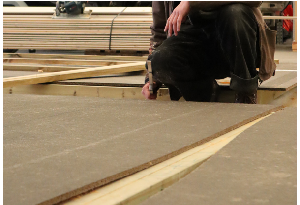
FIGURE 106. Adding of Hunton Intello Plus to walls
