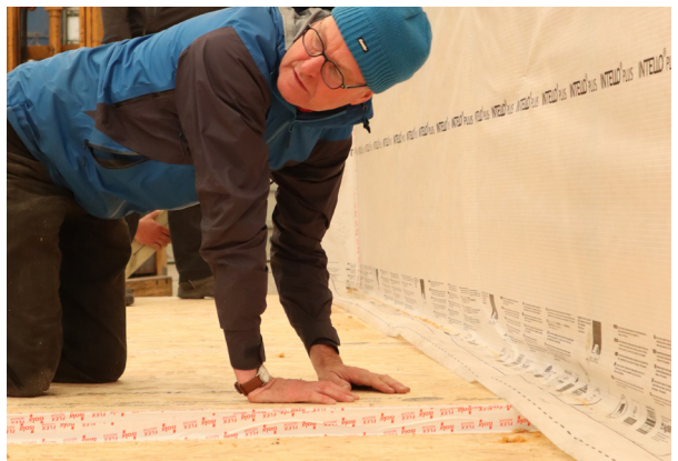
OSB was then added on top of the floor insulation.
