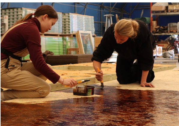
FIGURE 103. Painting tar and linseed oil mixture to floor base for waterproofing
