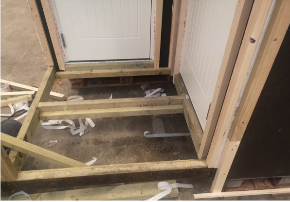
FIGURE 114. Frame of outdoor deck is added
