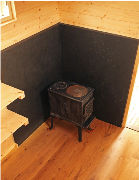
FIGURE 78. Final fire-protection solution (without glass plate)
