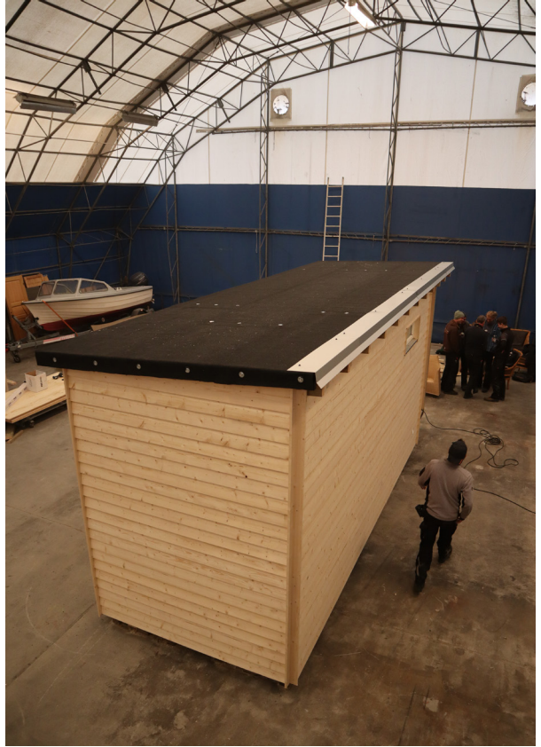
FIGURE 122. Custom metal roof flashing is installed along with bitumen-felt roofing
