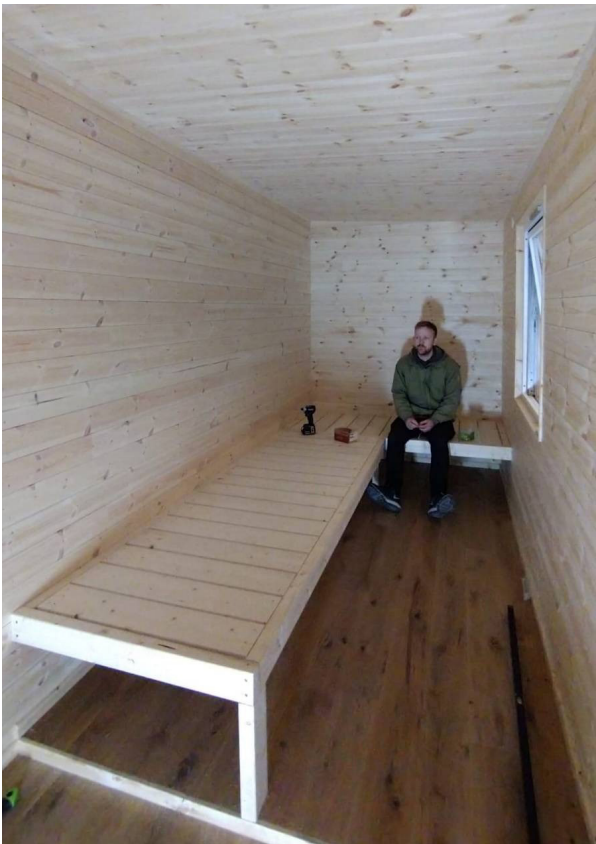
Furniture installation by Sami Rintala's carpenters.
