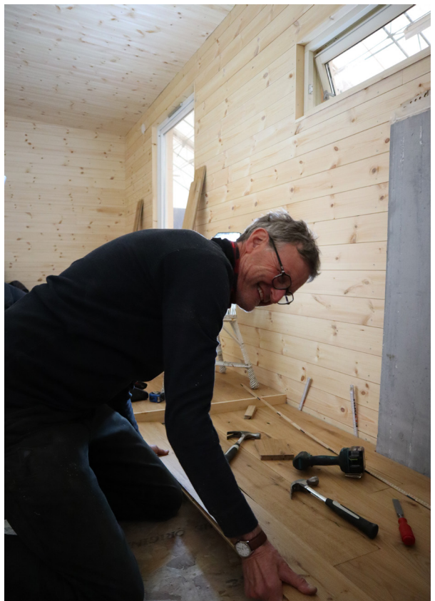
FIGURE 123. Installation of oak flooring
