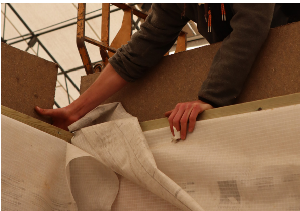
FIGURE 110. Screwing walls together
