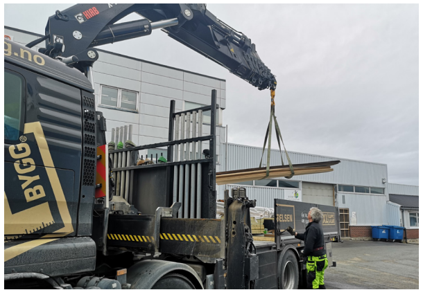
FIGURE 98. Material delivery by XL Bygg
