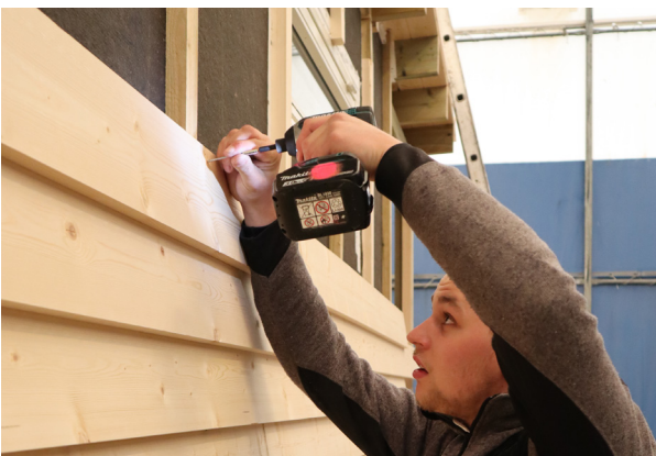
FIGURE 116. Exterior cladding is mounted
