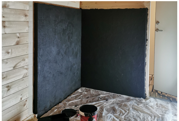
FIGURE 128. Fire-proof paneling after plaster and paint
