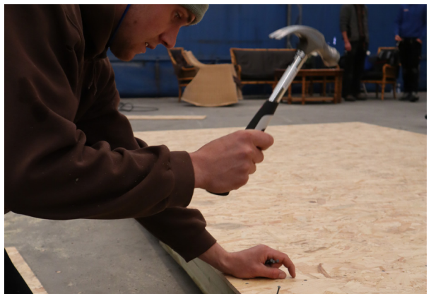
FIGURE 100. Adding OBS floor base
