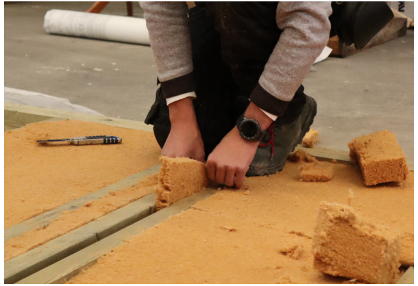
FIGURE 105. Adding of insulation to walls
