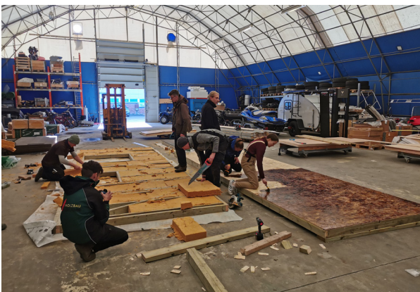
FIGURE 104. Simultaneous construction of floor and walls
