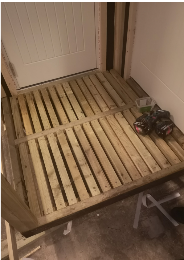
FIGURE 125. Decking from scrap materials is completed
