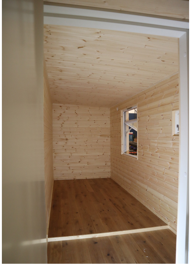
FIGURE 126. Finished interior cladding and flooring
