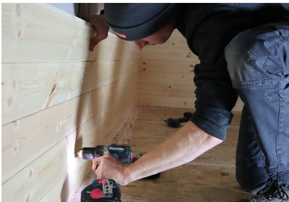
FIGURE 119. Interior cladding being screwed into place
