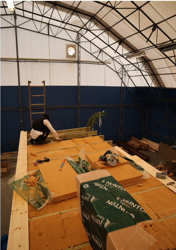
FIGURE 115. Insulation is added to the roof
