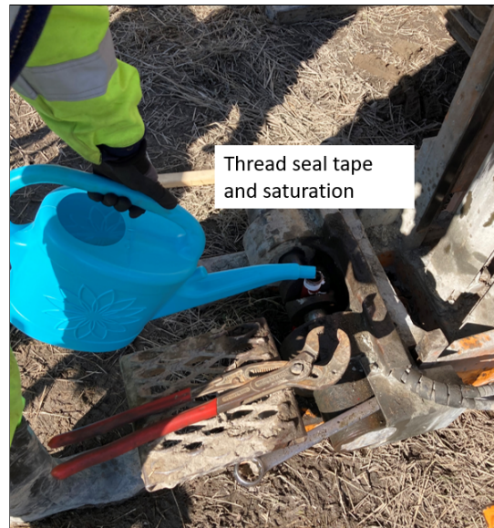
Figure 5.6: Installation procedure of water stand pipes
