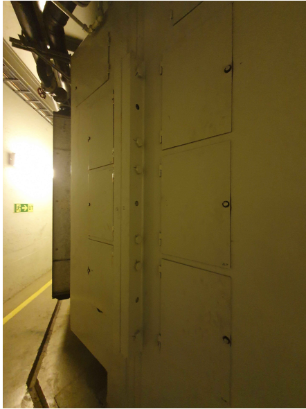
(a) Hatches through which field-joints were accessed. Sensors were installed at three vertical hatch levels.
