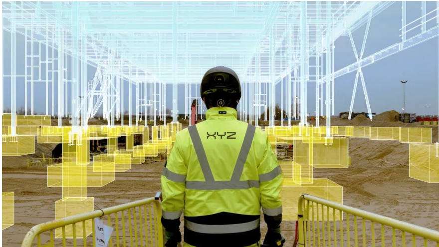
Figure 2.3: Illustration of XYZ AR system to project 3D models onsite. [23]
