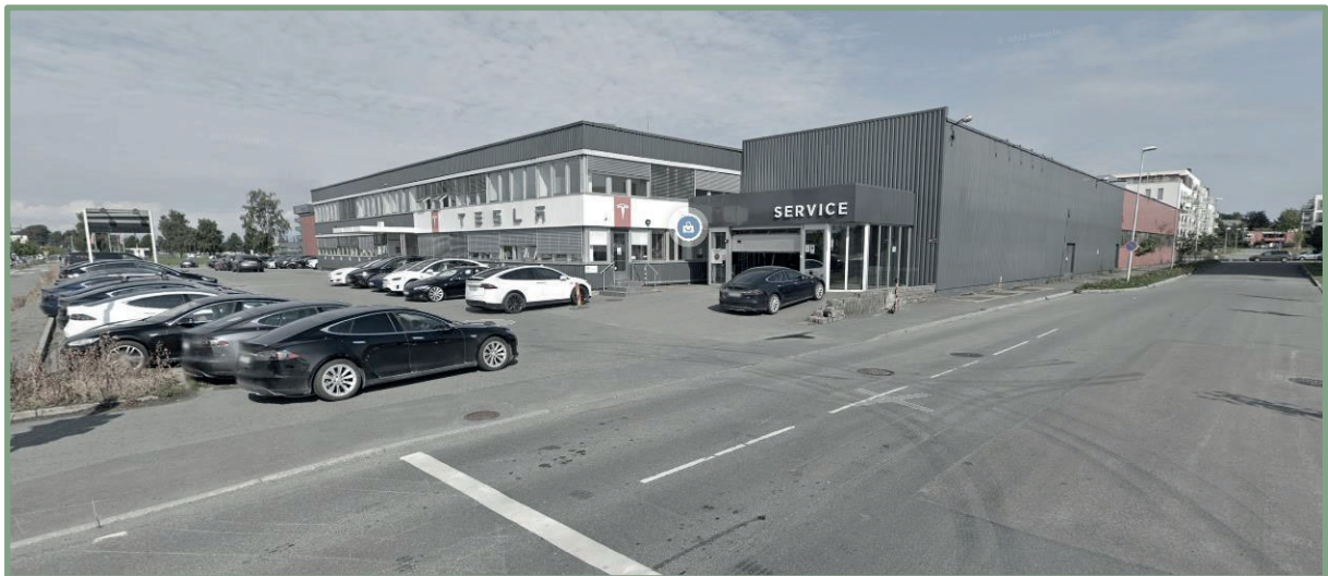
Figur 11: Tesla servicesenter Trondheim (Google street view, 2019).
