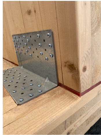
(b) Steel bracket side view
