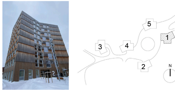
Fig. 2. Building layout at Moholt Student Village (right) and the view of Building 1 (left).
