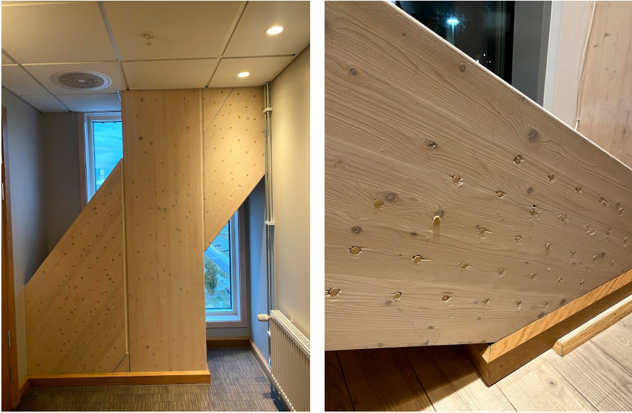
Figure 2.6: Connections in glulam truss
