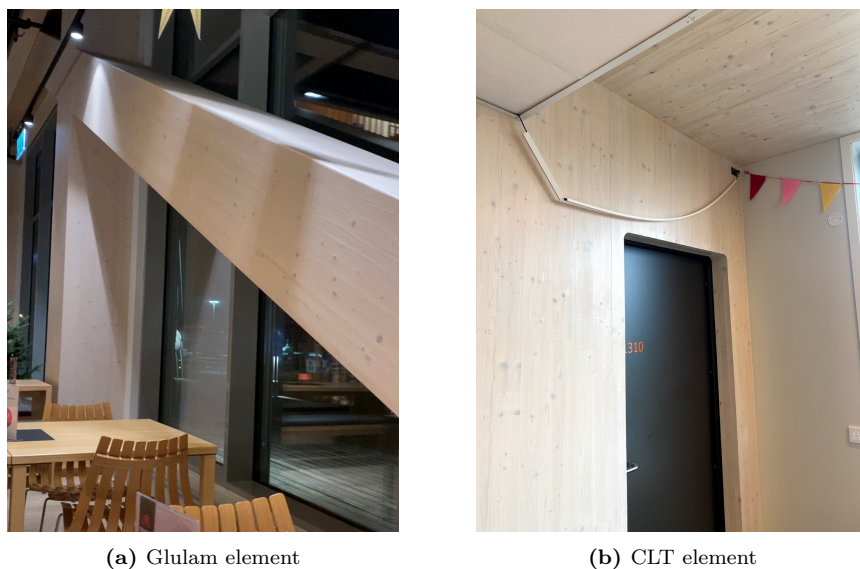
Figure 2.2: Examples of engineering timber products in buildings
