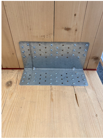
(a) Steel bracket with screws
