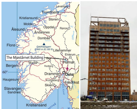
(a) Building location (b) The Mjøstårnet building view Fig.1. The Mjøstårnet building
